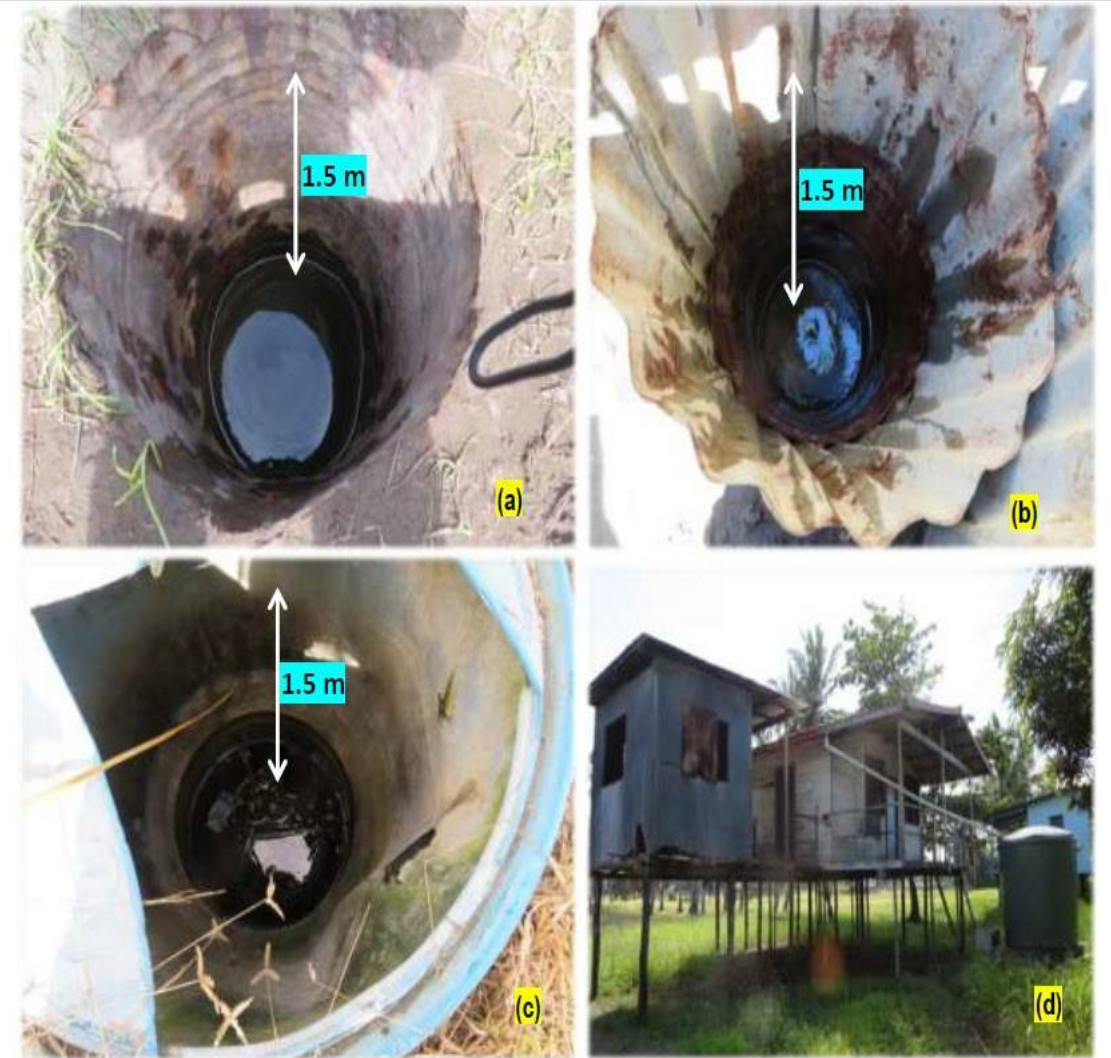
Figure 4: Current Manu Manu Village Water Supply System: (a) Shallow well at Manu Manu School. (b) Shallow well at the councillor's house at the village. (c) Abandoned shallow well at Kubuna School. (d) Staff house at Manu Manu School with a 2000 L tuffa tank for collecting rainwater.
